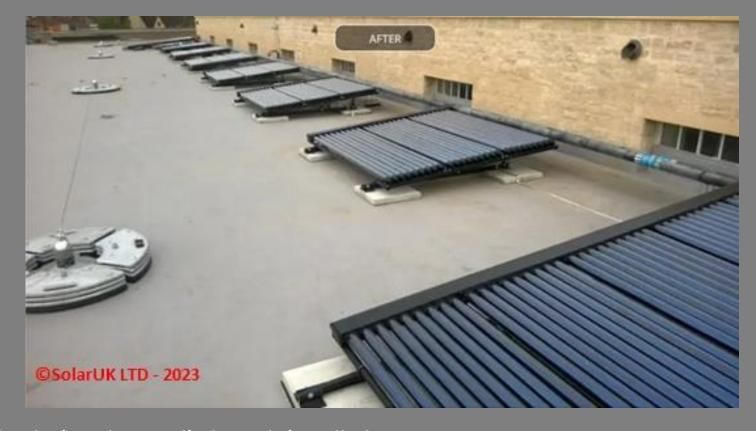
We designed, supplied, and installed 25m 2 of LaZer2 solar thermal collectors, feeding into the site's DHW infrastructure, providing 21MWh-th of hot water and reducing the reliance on gas. Our 3-man team led by lead LaZer2 installation engineer, Nick Martyn, and project managed by our Technical Director, Duncan Lee, installed and commissioned the system in c.6 weeks.
